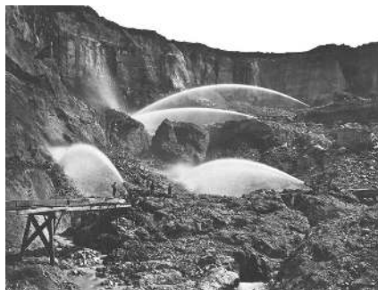
Figure 1.1: Hydraulic Gold Mining by Carlton Wakins is in the public domain - Hydraulic mining in the 1880s in Nevada City, California
