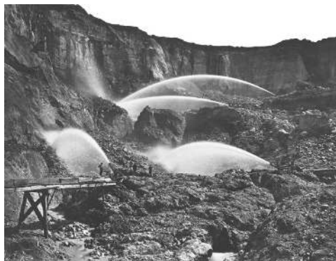
Figure 1.3.1: Hydraulic Gold Mining by Carlton Wakins is in the public domain - Hydraulic mining in the 1880s in Nevada City, California
