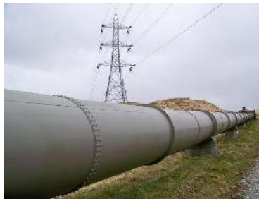
Figure 5.1: Pipeline by James T M Towill is licensed under CC BY-SA 2.0
